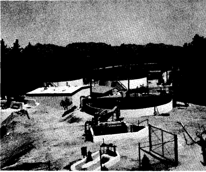
Lake Arrowhead Sanitation District Sewage Treatment plant. A typical small treatment plant providing primary and secondary treatment. Primary treatment to remove most of the sludge occurs in the structures in the foreground. Secondary treatment consisting of contact aeration and activated sludge takes place in the large tanks in the back.
