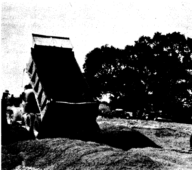
FIGURE 3 Off-site mixing is important. Then transport the soil mixture to the green.
