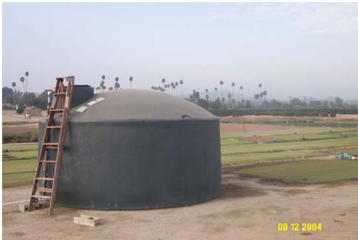
Recycled water was transported to the study site and stored in a 6000-gallon tank.
